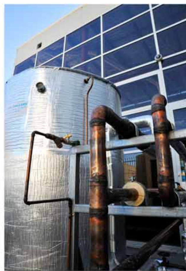
Buffer tank and chiller unit on site in Wyong
