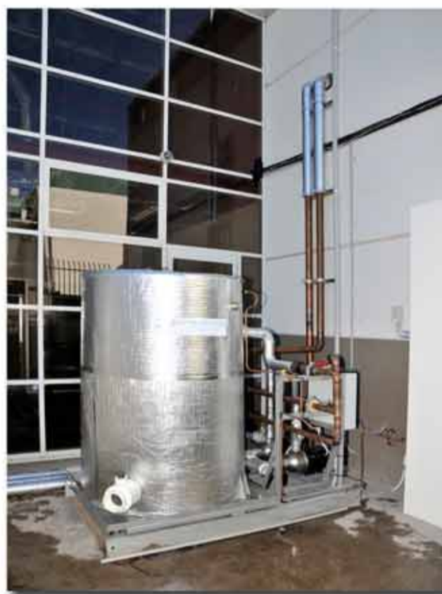
Buffer tank and chiller unit on site in Wyong
